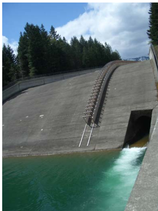
Cle Elum spillway with fish bypass (dry during visit)
